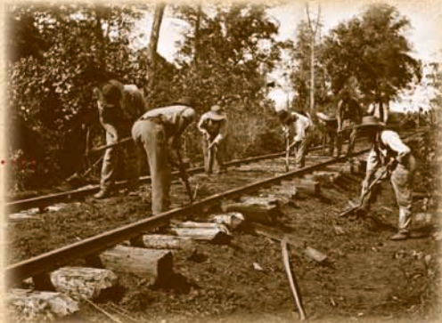
Men repair steel railroad tracks in 1863.
