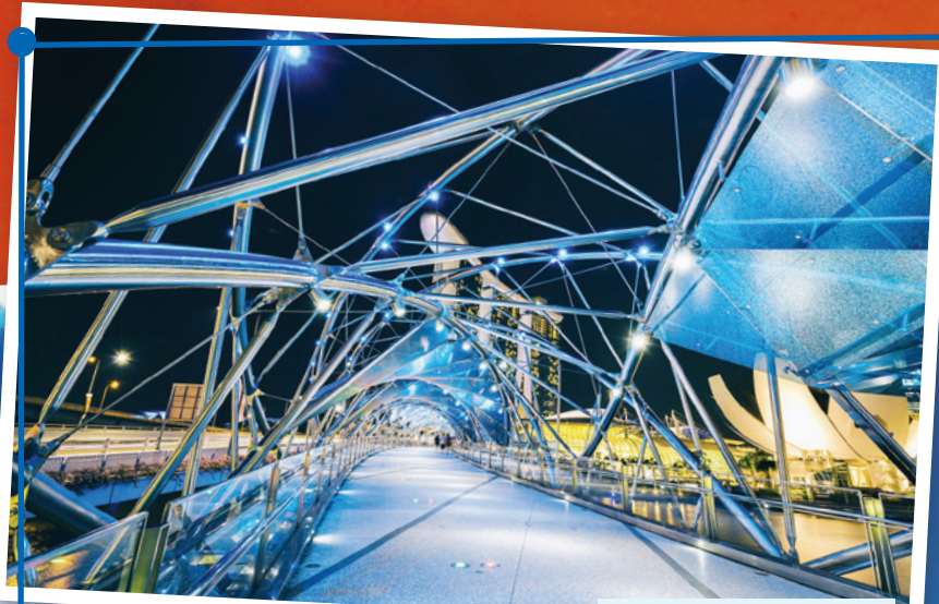
Helix Bridge's open design lets people see the city lights.
